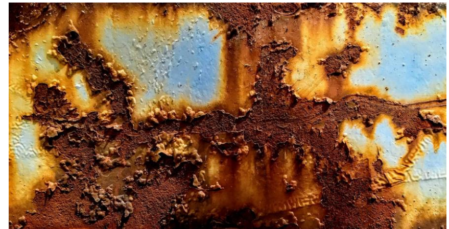
Bron: Corrosion & Metal Fencing - Diamond Fence (Aust) Pty Ltd
